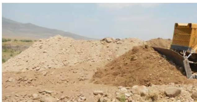
Figure 4-3-4.6 Mounded Sand-and-Gravels after Excavation
