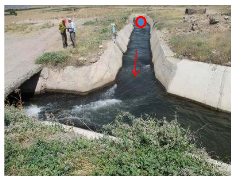
Figure 4-4-4.4 Outlet of Pipe from Arzni-Shamiram Canal (ø800mm) (Arzni-Branch Canal at No.25)
