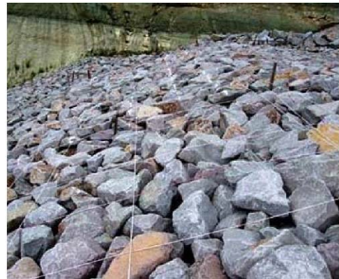
Figure 6-5-6.4 Example of Rock Rip Rap
